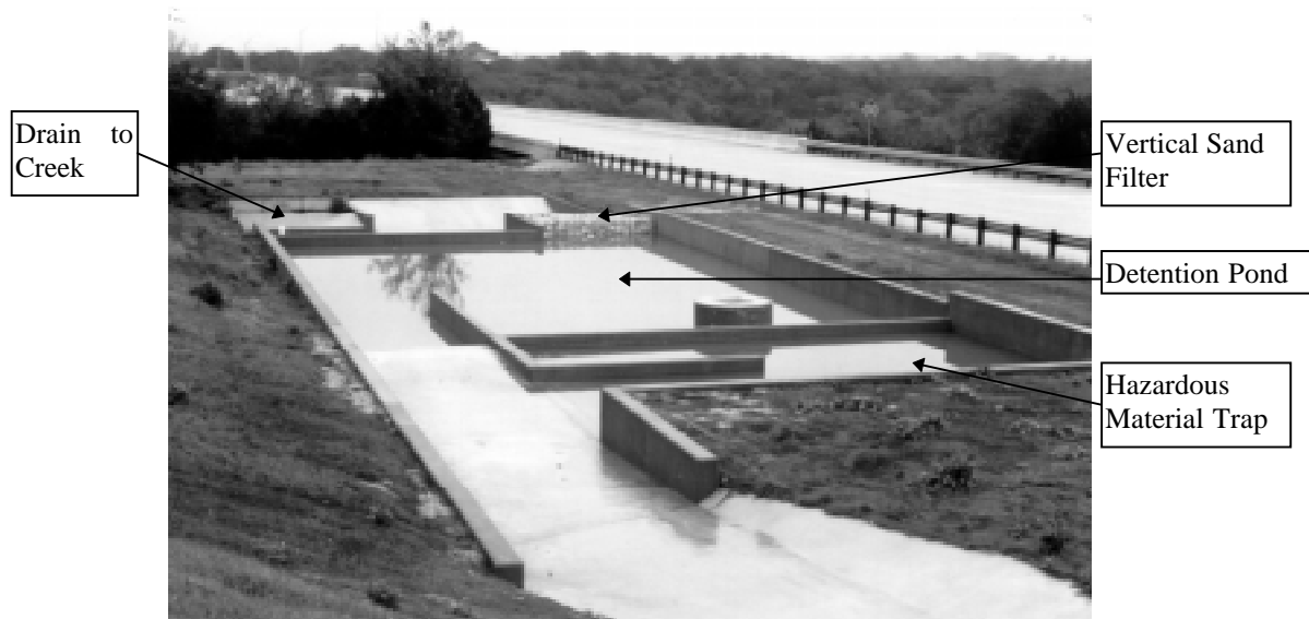
Figure 6.2 Typical Vertical Sand Filter System
